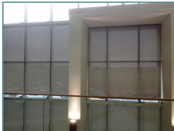
Screen roller blinds fully deployed
