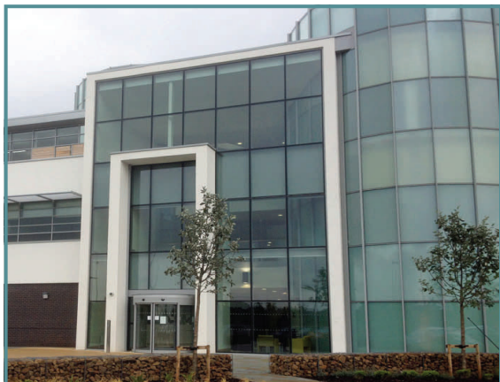
Full height glazing to reception area
