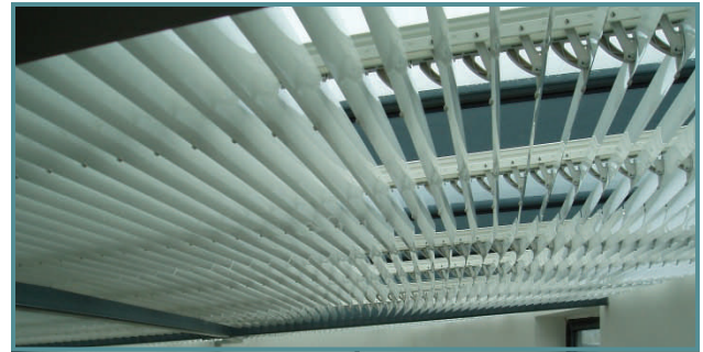
Close up of blinds at roof level
