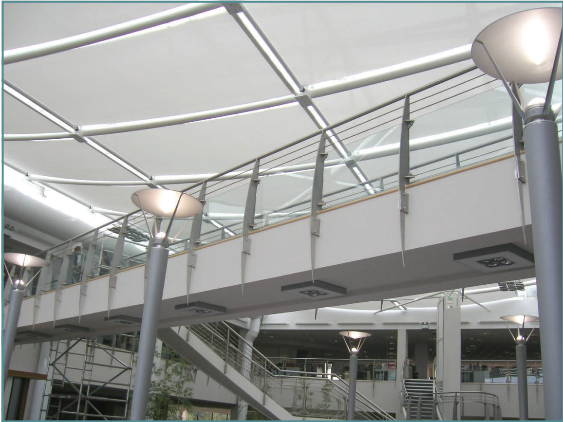
Blinds fully deployed over internal walkway
