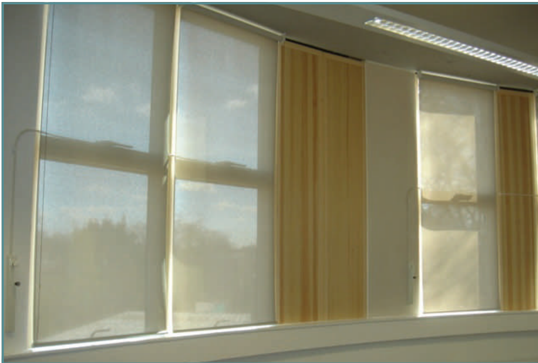
Blinds designed not to interfere with window actuators
