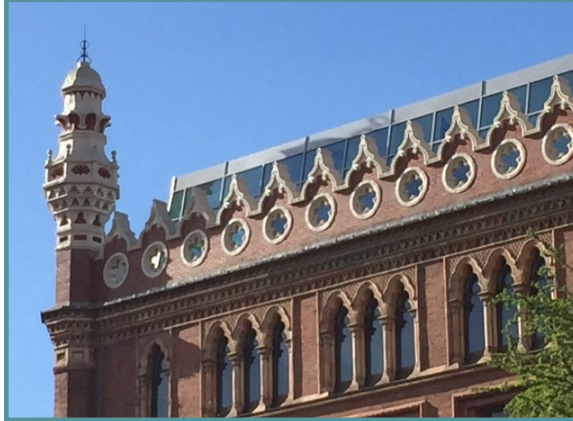
Sloping glazing on top floor
