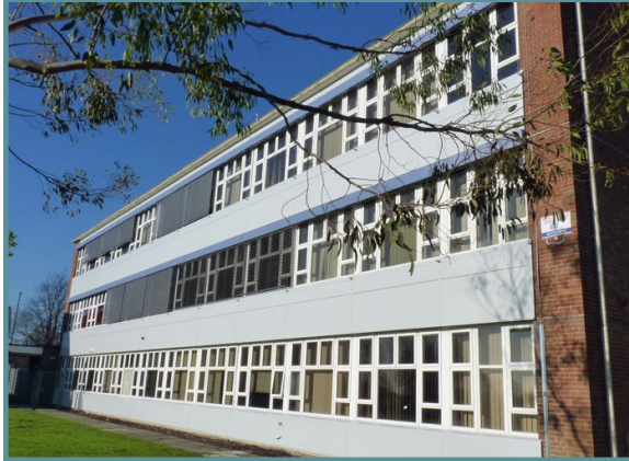
External venetians to 2 floors
