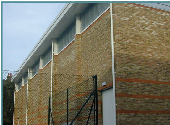
Rear elevation of multi-use hall
