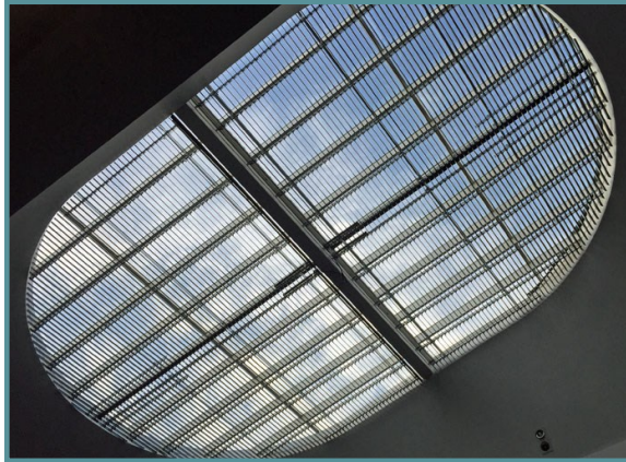
Rooflight blinds fully open
