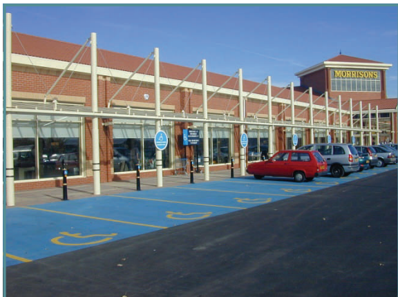
External view of blinds deployed
