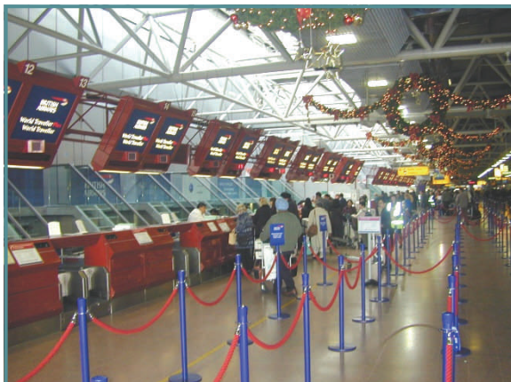
Blinds shade rooflight above check-in desks
