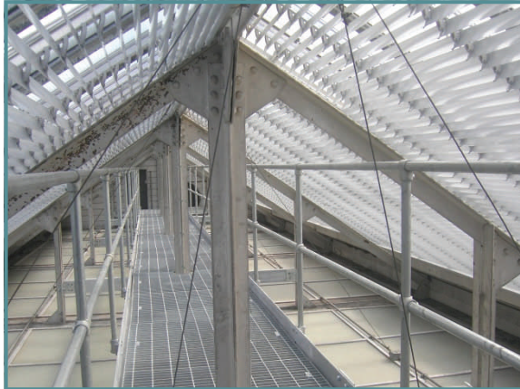
Blinds fitted above barrel vaulted ceiling
