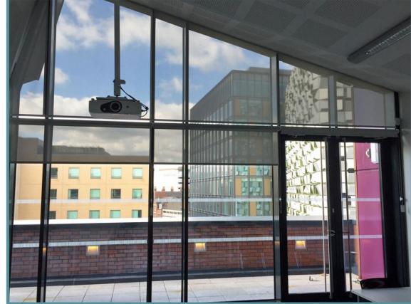
Screen roller blinds to curtain walling
