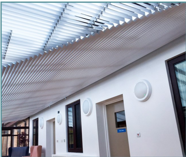
Louvres cut to match angle of glazing
