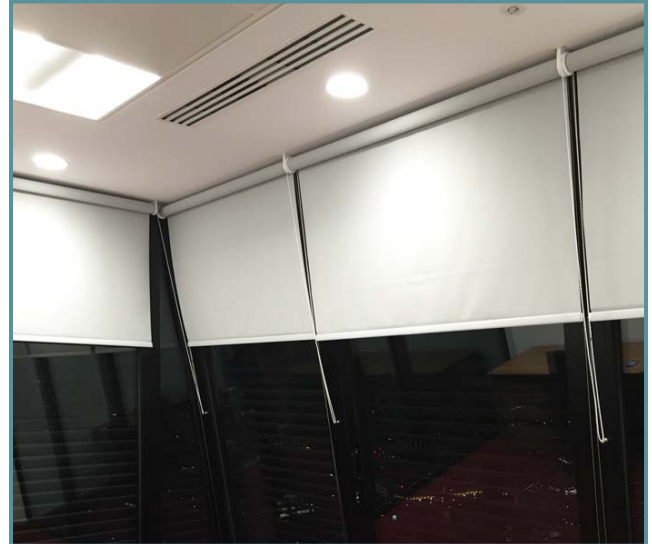
Operating chains retained on mullions
