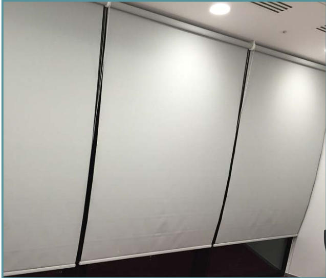
Blinds partially lowered on guide wires
